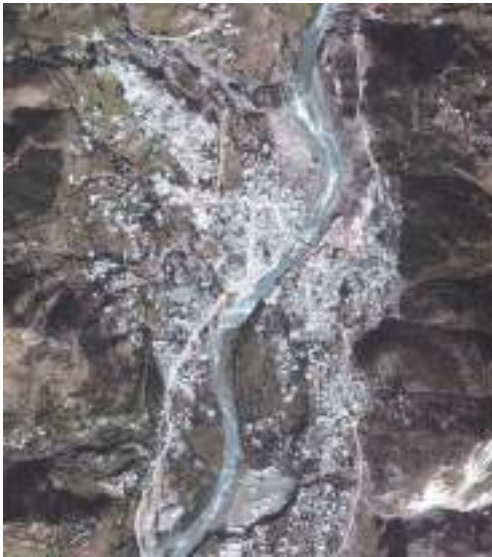
Figure 32.2 Satellite image showing destruction of a bridge as a result of flood.
